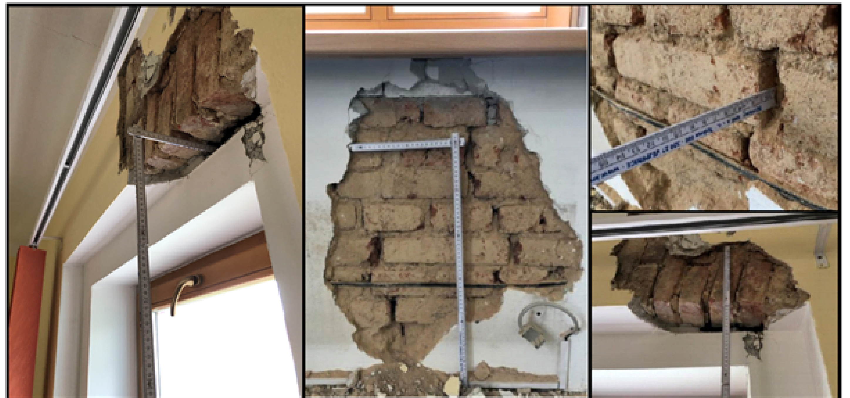
The probe in the window sill and lintel on the 2nd floor of the building east wing.
