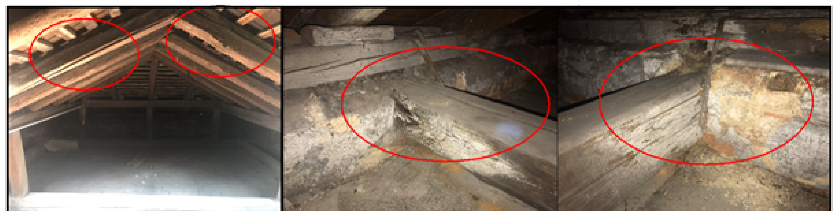
The extent of wooden truss elements damage
