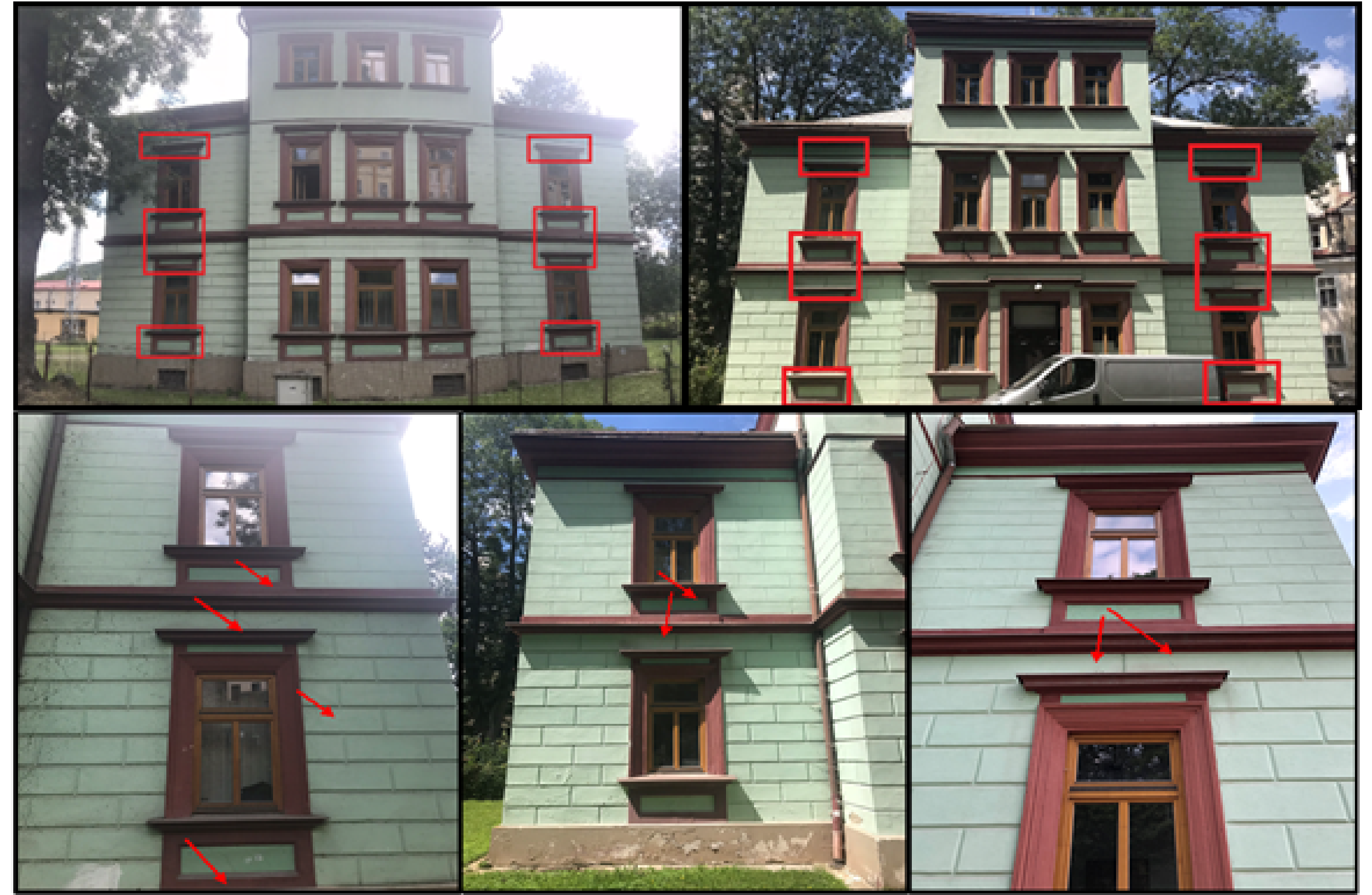
The western and eastern facades of the building with the marked places and direction of the cracks.
