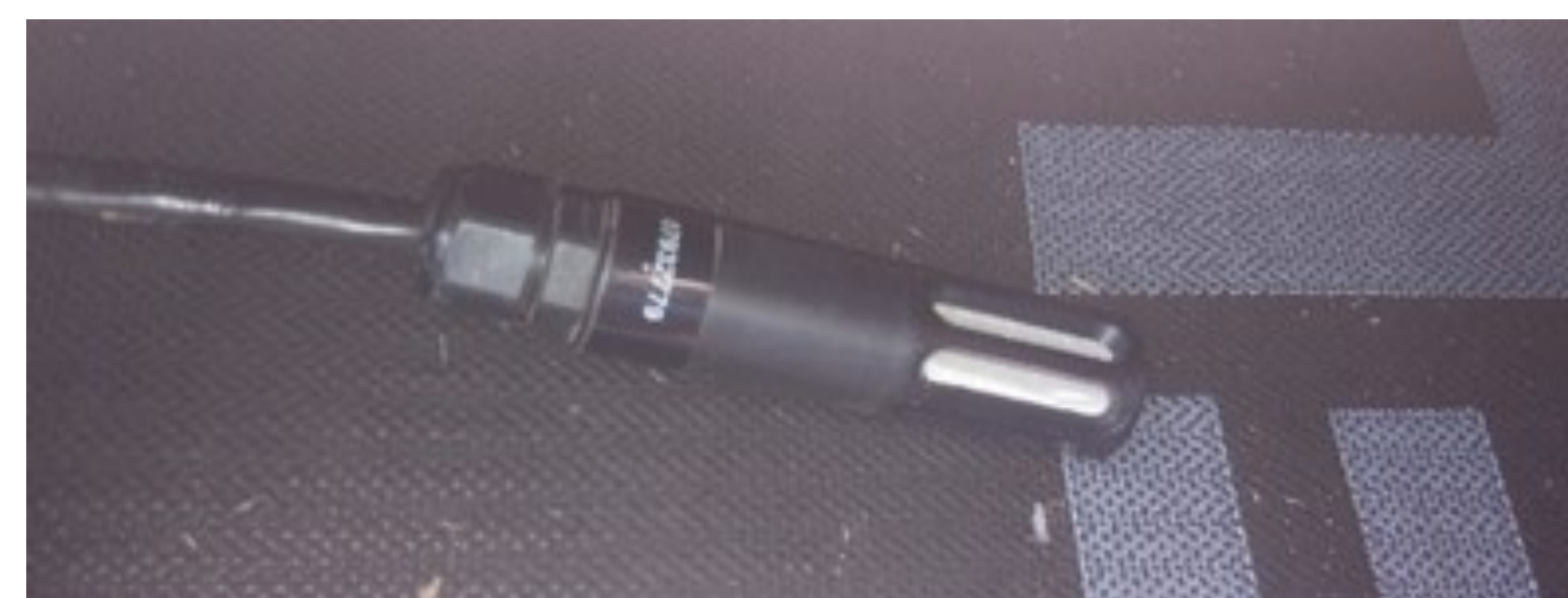
Figure 1. Thermal-humidity sensor installed in air cavity [7]
